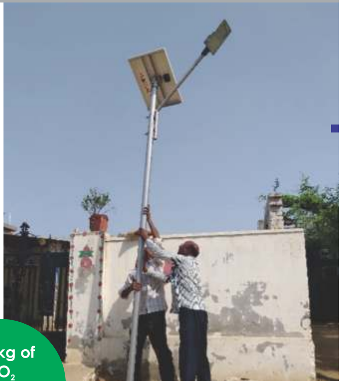
Glimpses of solar street lights being set up
